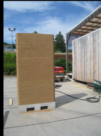
The wall is finished
